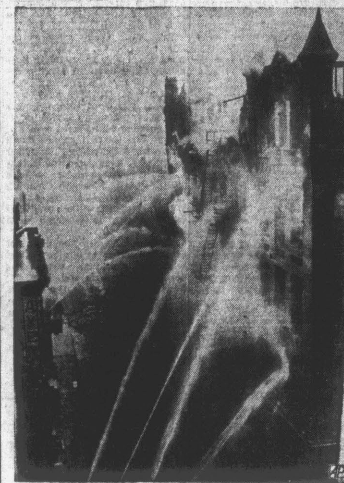
Firemen play streams of water on flames sweeping through a downtown warehouse in Philadelphia. Damage was estimated at $1,000,000. Debris from a crumbling wall fell on a fire engine and injured three firemen. The falling wall also hit a live trolley wire which fell across another engine, charging it with electricity. Three hundred firemen from 40 engine companies fought the flames for four and a half hours. (AP Wirephoto).
