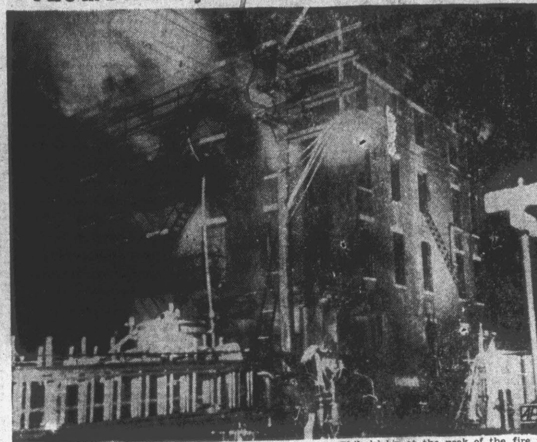
Flames burst from windows of a dormitory for homeless men at Philadelphia at the peak of the fire in which six are known to have perished. Ten others were reported missing, and at least 38 were injured. The dormitory was operated by Volunteers of America, Inc. It housed 66 men, many of whom were employed as street corner Santa Clauses. (AP Wirephoto).
