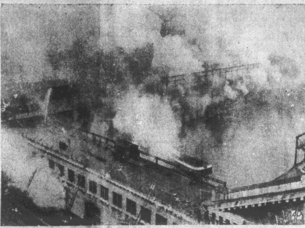
A great cloud of smoke rises from the Grace Line's pier 57 on New York City's North River waterfront during a fire that caused damage estimated by fire officials at more than $5,000,000. The flames started under the pier (upper left), spread through the building (lower left), connecting it with Pier 53 (not shown), where a liner was berthed. Fifty firemen suffered minor injuries. (AP Wirephoto).
