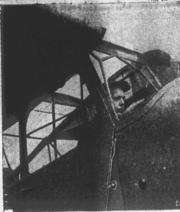
NEW LIAISON PLANE —Added window area to increase three-way visibility and a special door which may be jettisoned are features of this high-wing Aeronca 7BC monoplane ordered by the U. S. Army for liaison use.
