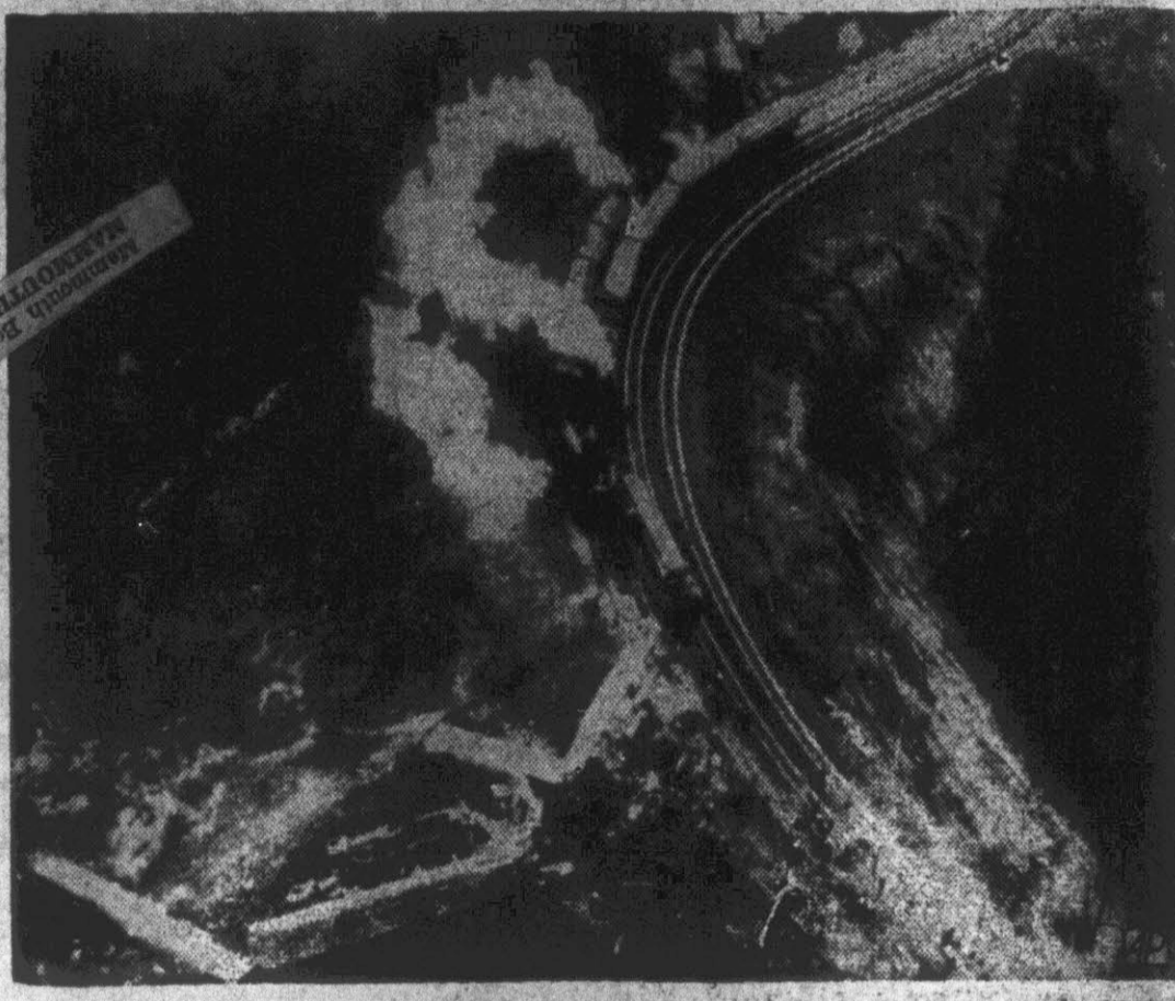
On a steep bank beside sharp "Benning Curve" near the Pennsylvania railroad's better known "Horseshoe Curve" the wreckage of the fast Detroit-to-New York passenger train, the "Red Arrow," left the rails a short distance from Altoona, Pa., killing 22 persons and injuring about 100. Smoke puffs come from a salvage train directly behind one of the "Red Arrow's" cars still on the road bed. (AP Wirephoto).
