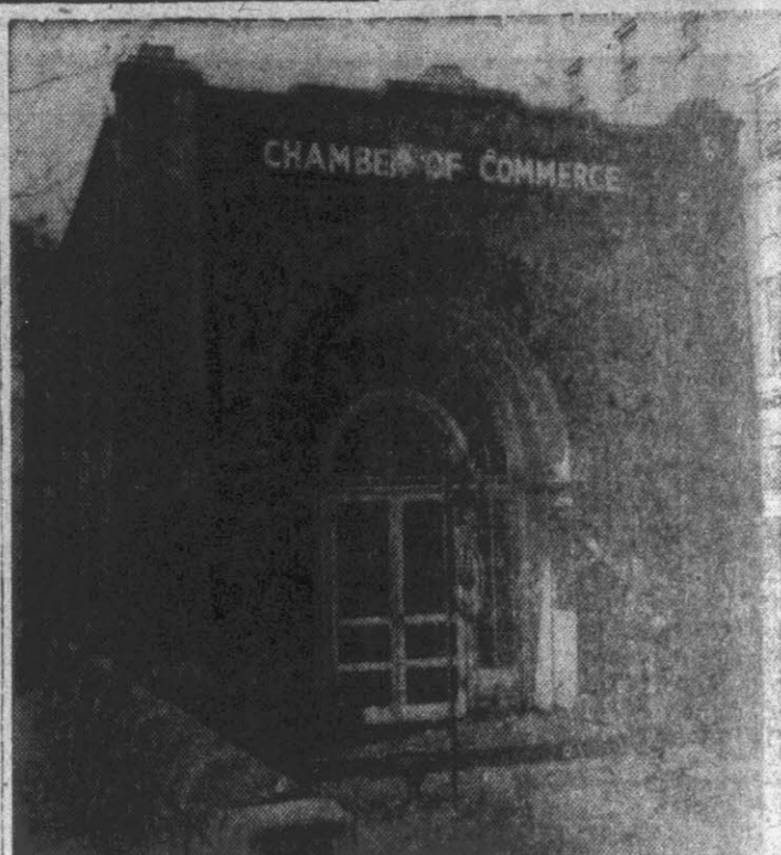
HOUSE OF COAL —The Chamber of Commerce building at Williamson, W. Va., is built of solid bituminous coal. Miners and operators joined in raising the structure in 1933.
