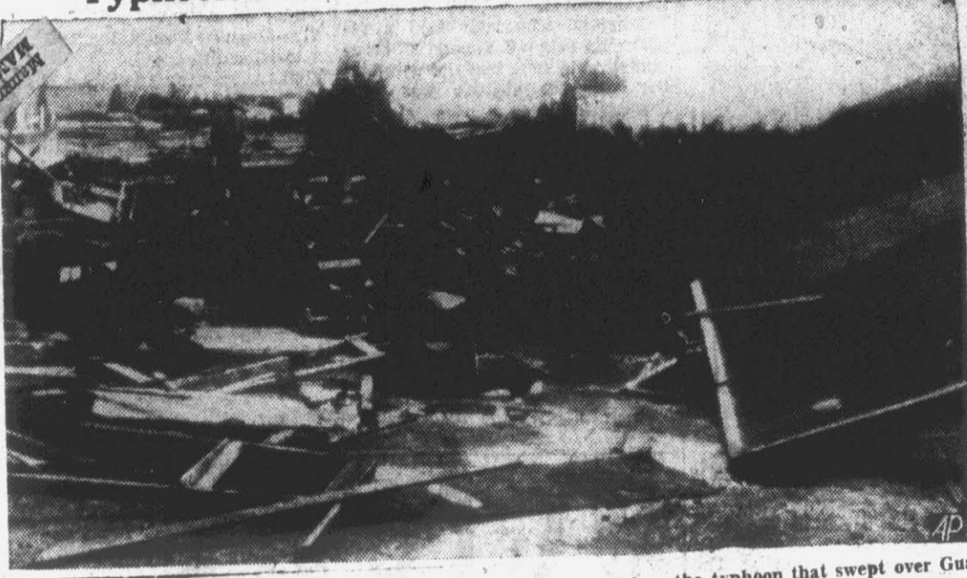
Spectators stand amid wreckage of pre-fabricated houses destroyed by the typhoon that swept over Guam island in the southwest Pacific September 21. The building in the foreground had housed headquarters of the 20th U. S. Air Force. (AP Wirephoto from 20th Air Force).
