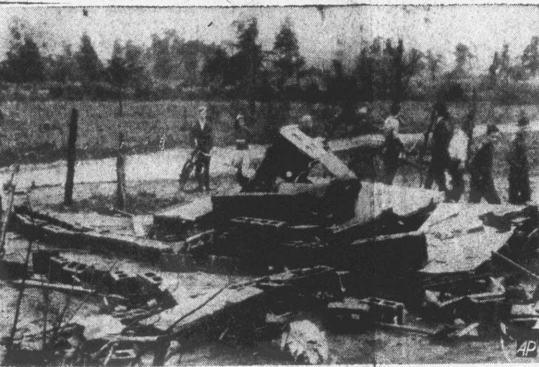
Little more than the foundation of the Nelson Jones home at Objibway, Ontario, remains in the wake of the tornado which swept across the Detroit river from southern Michigan. Three members of the Jones family were killed, and four others were injured, two critically. Two others escaped unhurt. Many other buildings in the area suffered like fate. (AP Wirephoto).
