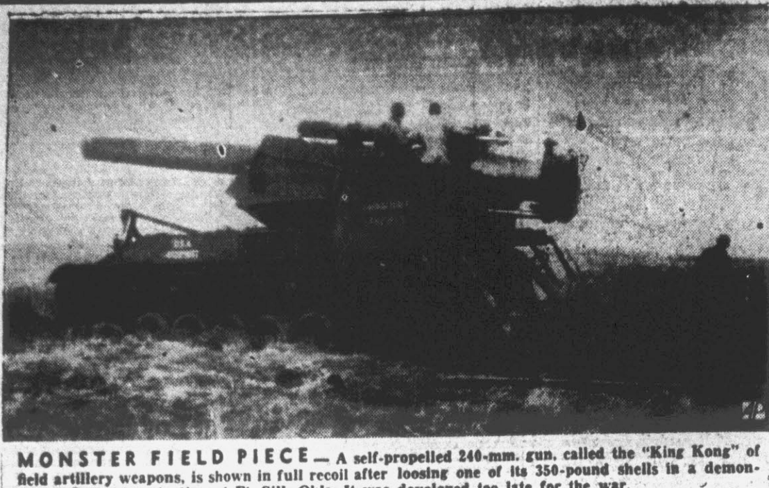
MONSTER FIELD PIECE—A self-propelled 240-mm. gun, called the "King Kong" of field artillery weapons, is shown in full recoil after loosing one of its 350-pound shells in a demonstration at Ft. Sill, Okla. It was developed too late for the war.
