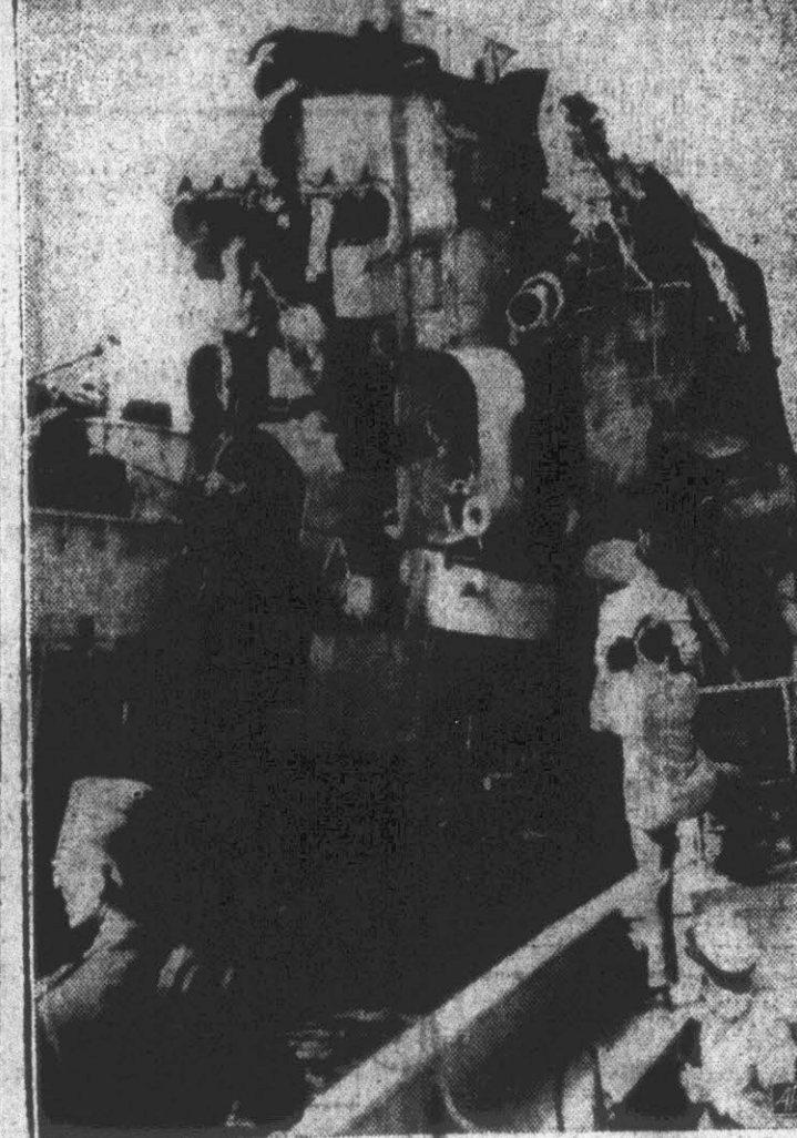
This mass of twisted wreckage was left by three explosions which ripped through the U. S. S. Solar, naval destroyer escort, as she lay alongside a pier at the navy's huge ammunition depot at Earle, N. J. The deck and bridge have been twisted into an upright position. Five crew members were reported missing and 150 were injured. The Solar is a total loss. (AP Wirephoto)
