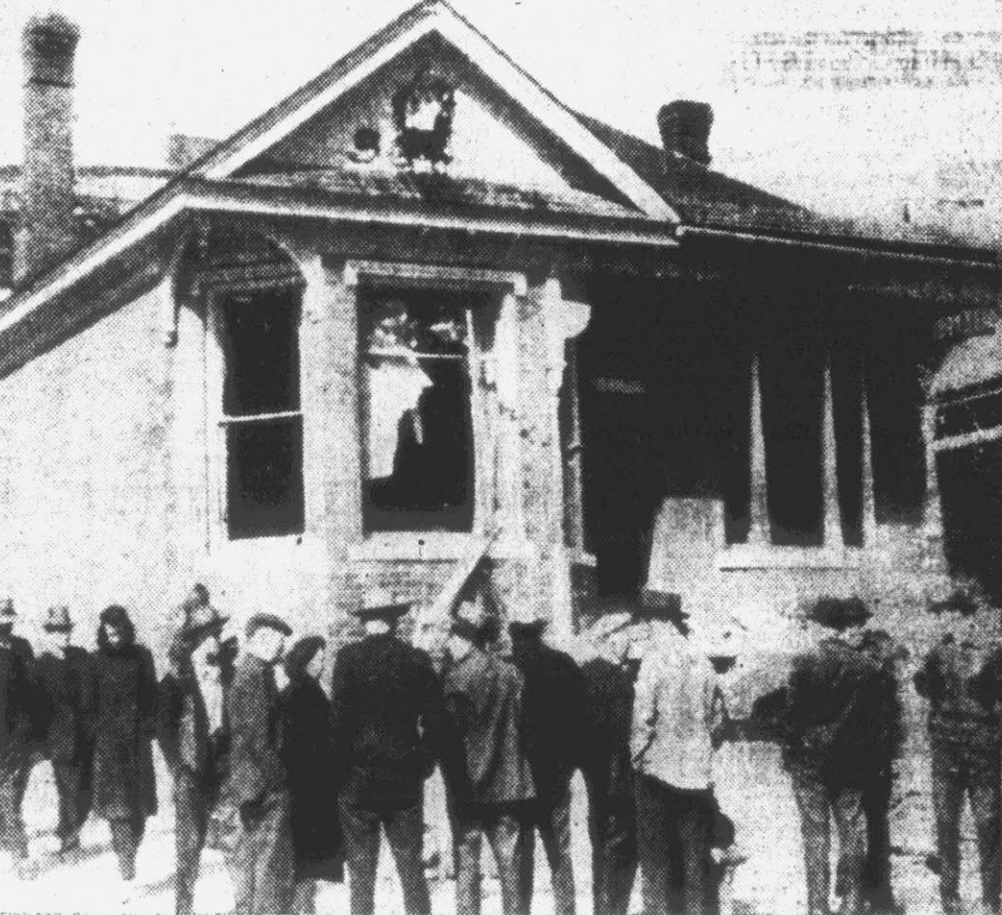
This house at 701 East Park street in Butte, Montana, was left in this damaged condition by a mob which has wrecked scores of buildings occupied by workers who did not join a miners' strike. The roving mob smashed doors and windows, chopped off porch supports, and invaded homes to smash mirrors, glassware, dishes and furniture. (AP Wirephoto.)
