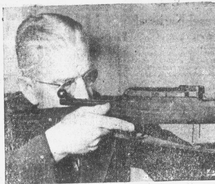
BOOBY-TRAP SOUVENIR? —A souvenir German semi-automatic rifle (Gewehr 41M) with a faulty "interrupter" is shown by Lovell Pace, Winchester gun engineer, to show how the weapon's bolt, if fired, could kill or maim the user. Experts believe faulty parts may have been weakened intentionally by Germans to transform abandoned guns into booby traps.
