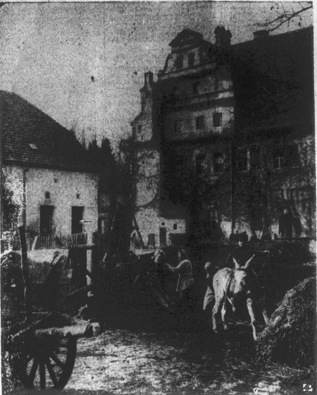
GERMANS IN NEW HOMES—German women tell in the farmyard of their new home (background) near Dresden, one of several estates the Russians have divided among workers.
