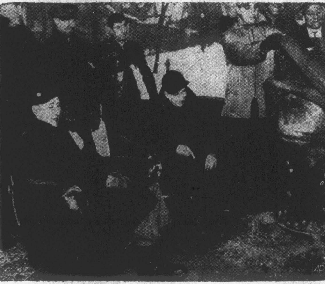
Two pickets relax in easy chairs in front of a gate to the strike-bound plant of the Bethlehem Steel Company at Lackawanna, N. Y., as a fellow picket tries to coax a little more heat out of a salamander while biting winds from Lake Erie whistle overhead. The other men also are pickets. The strike at the plant has kept 11,000 workers idle for nearly a week. (AP Wirephoto).
