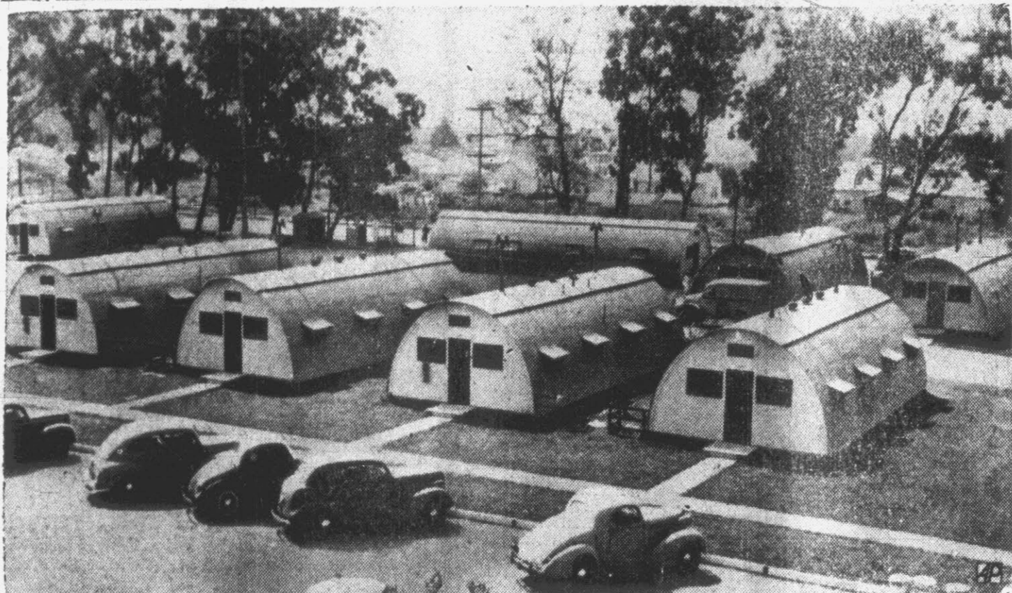
EMERGENCY 'QUONSET' HOUSING—These Quonset huts, converted for civilian use during the housing shortage, were set up at Port Hueneac, Calif. They are insulated, have living room, two bedrooms, bath and kitchenette.
