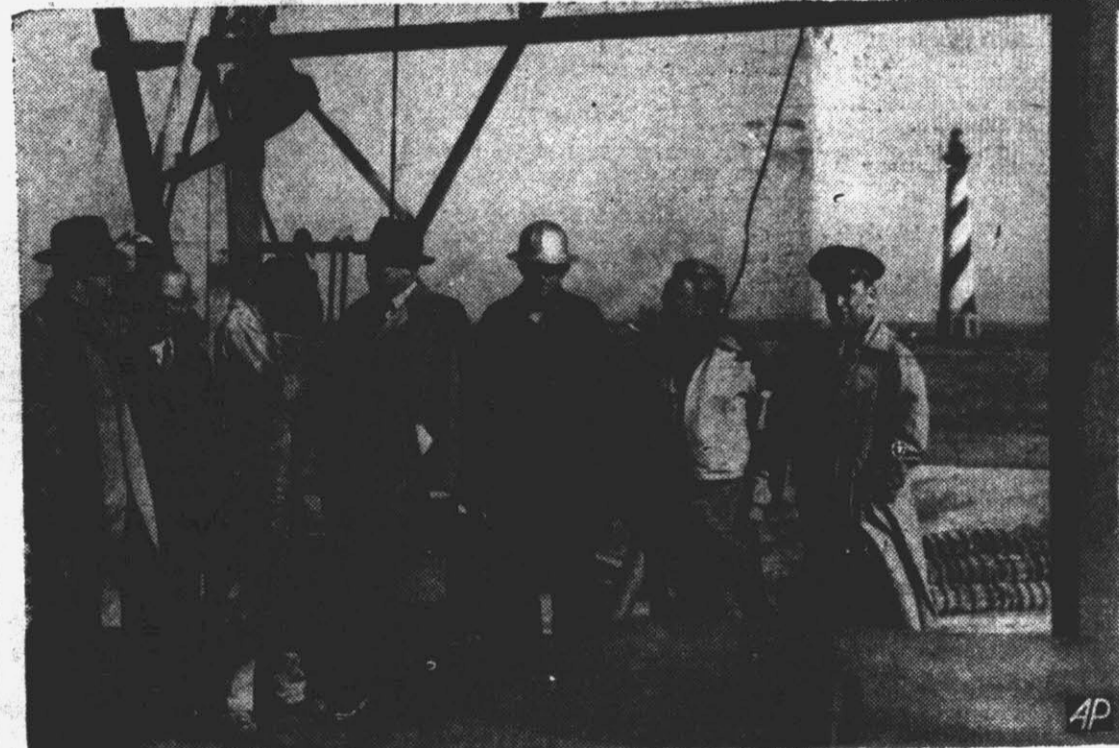
Against a backdrop of the oldest and tallest light house in America, the Standard Oil company got under way with drilling its first exploratory well on two million acres of land under lease in North Carolina. The scene is at Cape Hatteras a few minutes after drilling began. Right to left: Col. R. W. Lookridge, engineer of the war-time Canon project; Lloyd Noble, president of the Noble Drilling company; L. V. Fugener, driller; Oscar C. Schorp, president of the Carter Oil Company; 'Spit' Miller, project superintendent; K. D. White, Standard Oil geologist who directed the research prior to locating the well, and is now general director of operations, and M. A. Wright, chief engineer for the Carter Oil Company, a Standard subsidiary. (AP Photo).
