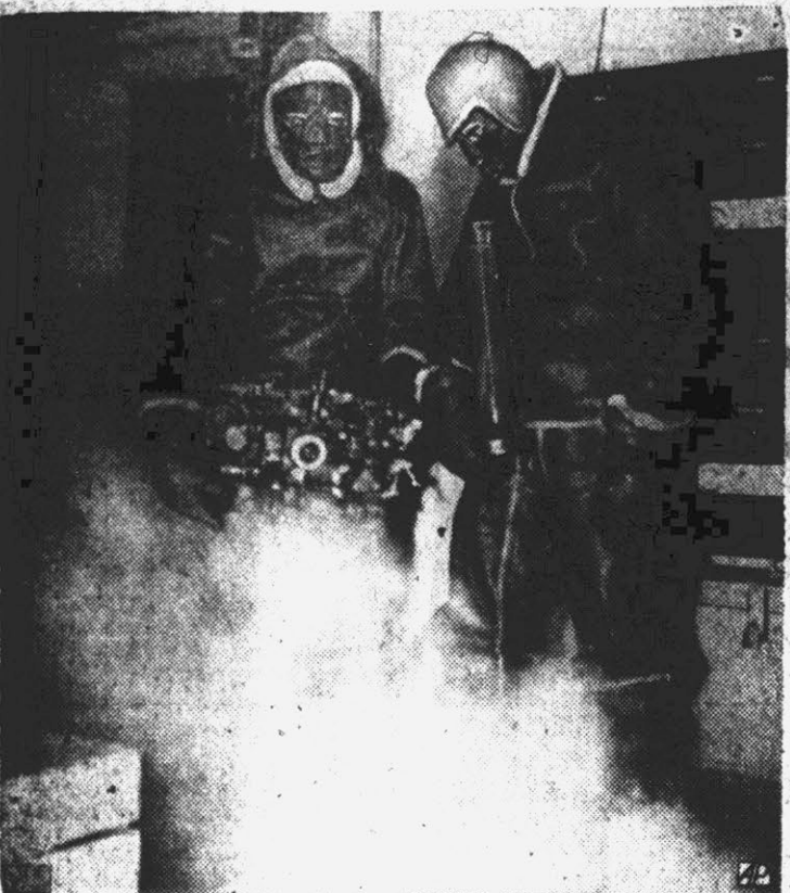
MEN FROM MARS —Bendix Aviation technicians wear masks and flying suits to ward off frostbite while checking high altitude performance of carburetors in a refrigerated "air box," which simulates temperatures as cold as —80 degrees.
