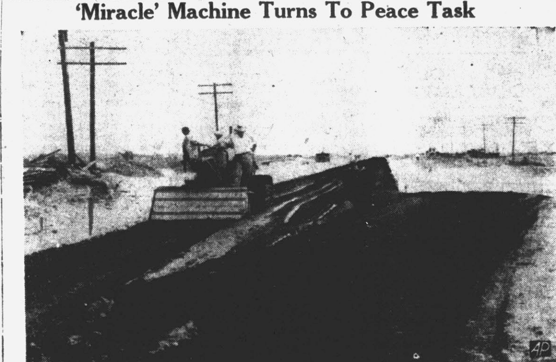
'Miracle' Machine Turns To Peace Task—Displacing an asphalt mixing machine and a whole fleet of trucks, this simple piece of machinery, developed and widely used during the war has been turned to the peace-time job of building a highway to Cape Hatteras on the North Carolina "Banks." The machine mixes asphalt and sand right on the spot, and lays the paving, 18 feet wide, at the rate of 4,000 feet in three days. Highway engineers in the distance watch with amazement. (AP Wirephoto).
