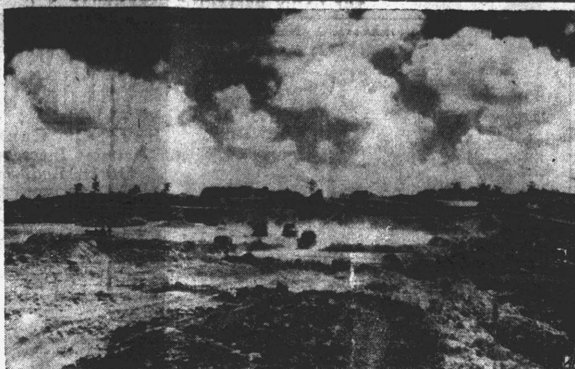
OKINAWA AIRFIELD GROWS—Trucks and hand shovels and bulldozers to construct an airfield on Okinawa which will serve as a base for attack on Japan.
