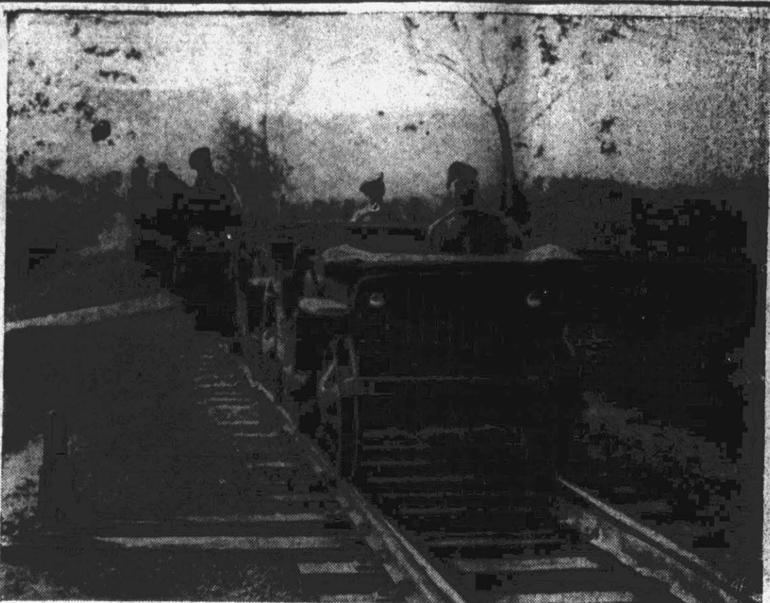
JEEP RAILROAD —Indian engineers built this rail supply line through liberated Burma. Using automobile power, it's called the Myitkyina Southward Jeep Railway.
