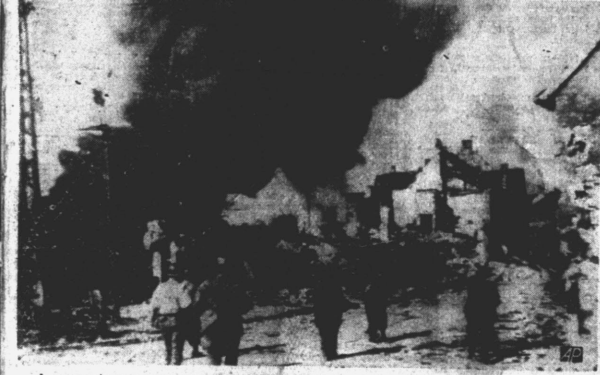
A reconnaissance group of the 63rd Division walks cautiously through the wreckage in the streets of Saarbrücken, Germany, six kilometers from Saarbrücken. The thick column of black smoke in background was not explained in the caption received with the picture. (AP Wirephoto via Signal Corps radio).
