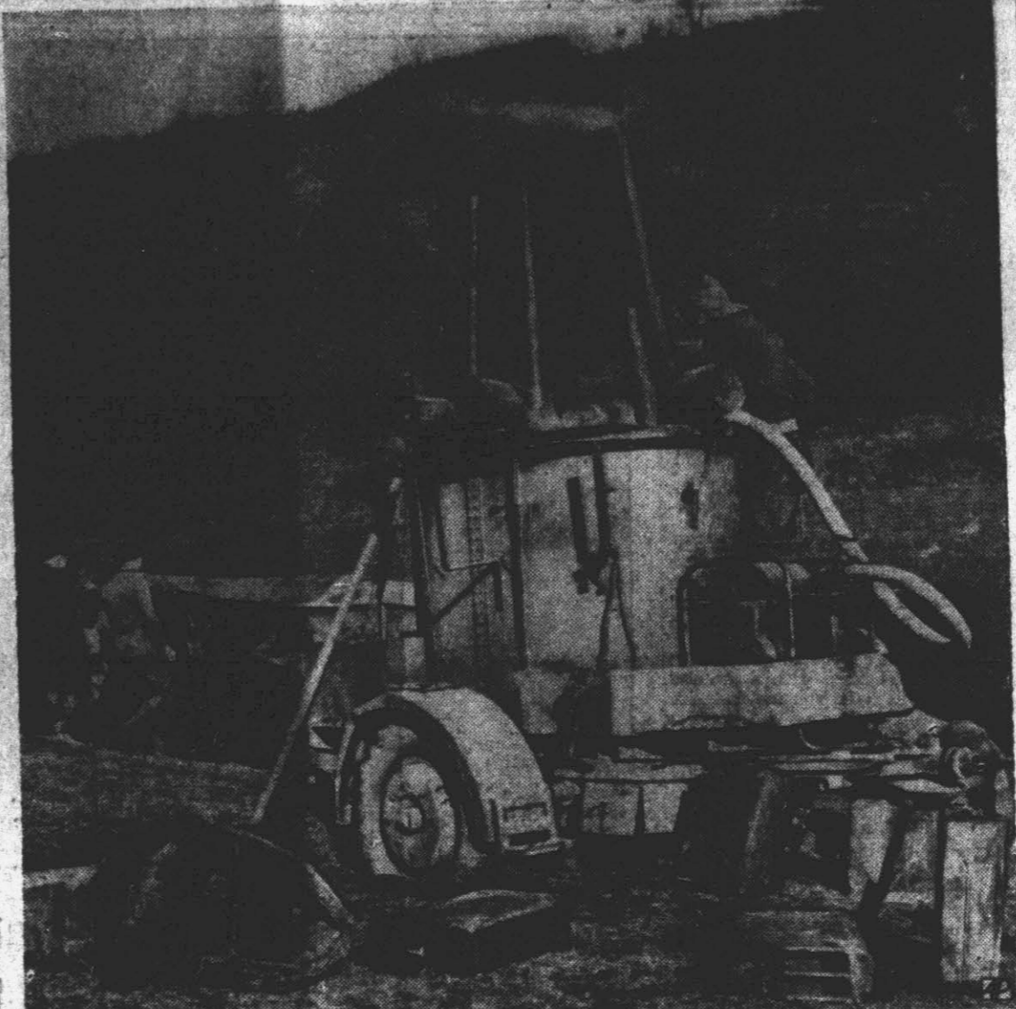
INGENIOUS PLUMBING —It looks a little like an anti-aircraft emplacement, but actually it's a field shower built of captured German materials by Yanks in Luxembourg.
