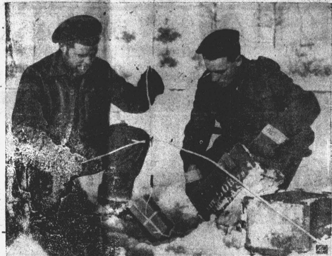
DYNAMITING FROZEN CANALS —Cpl. F. W. Brown of Rexton, N. B., and Sapper W. A. Guerdard of Sudbury, Ont., lower explosive charges through holes cut in the thick ice of a canal near Nijmegen, Holland. The ice is blasted to prevent enemy crossings in efforts to penetrate Canadian lines during the cold weather.
