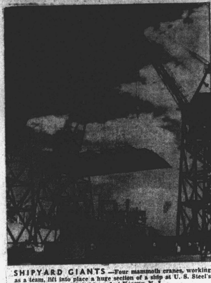
SHIPYARD GIANTS —Four mammoth cranes, working as a team, lift into place a huge section of a ship at U. S. Steel's Federal Shipyard at Kearny, N. J.
