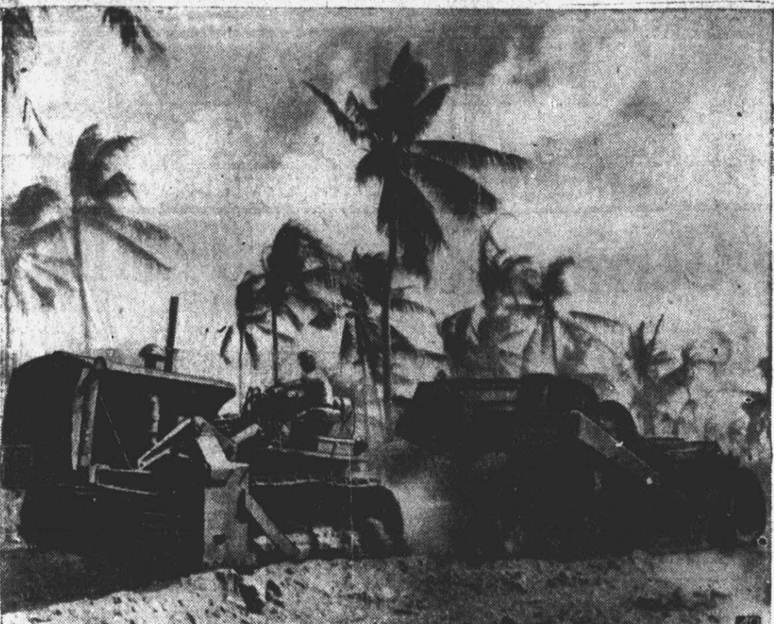
BUILDING AN AIR STRIP —The operator of a Navy construction battalion (Seabee) machine levels off ground for an air strip on a unidentified tropical island.
