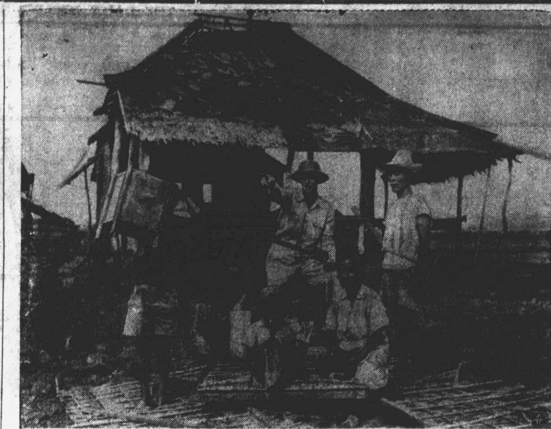
MAKING WAY FOR AIRSTRIP — Lt. Victor P. Roberts of the U. S. Engineers describes proposed Mindoro island airstrip to Filipino family being evacuated from site.
