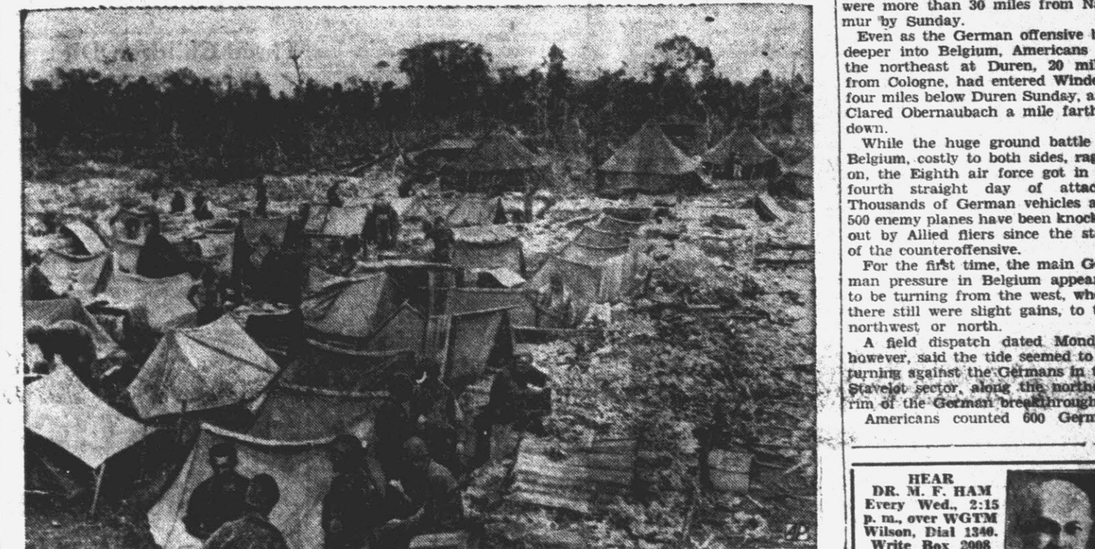
PALAU STREET SCENE —Seventh Army Air Force men set up housekeeping in tents on the site of demolished Jap installations in the Pacific Palau islands.
