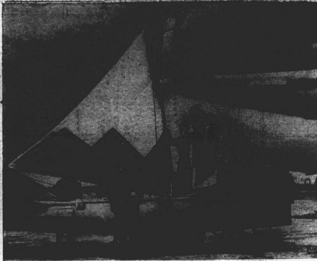
DESIGNED FOR AIR-SEA RESCUE—RAF plane erect an airborne lifeboat which is designed to be dropped by parachute. Twenty-seven feet long, it has sails, two motors.
