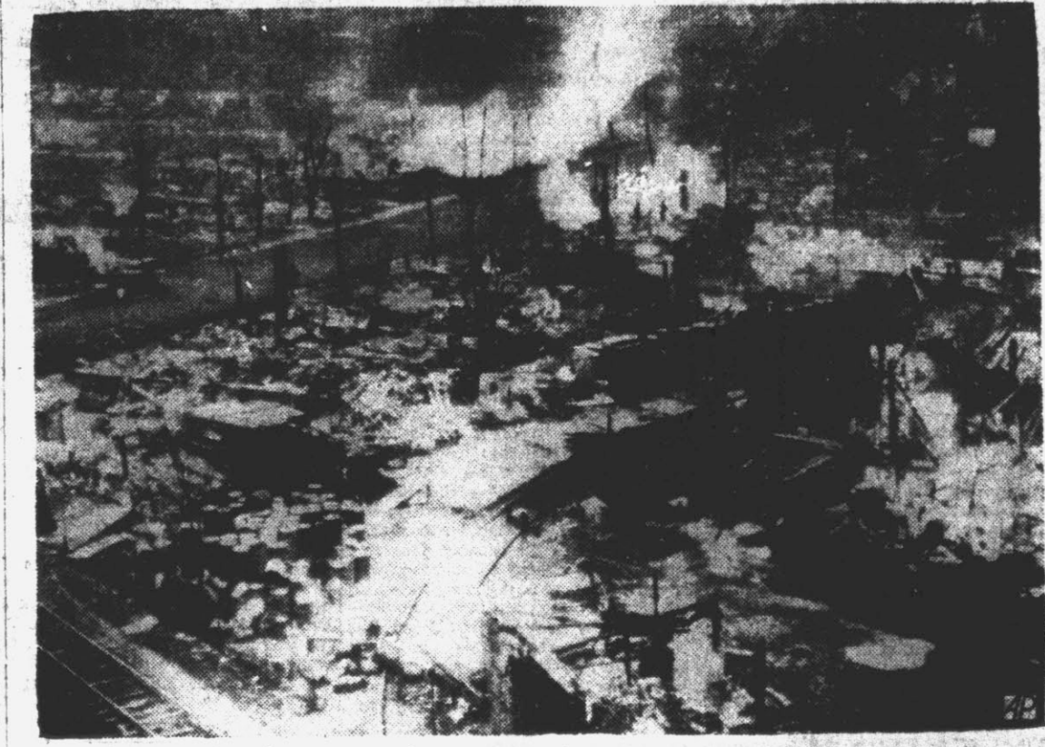
A multi-million dollar blast, following the explosion of two gas tanks, left only the framework of dwellings and burning debris in the surrounding area in Cleveland. More than 3,600 persons were left homeless, and at least 114 were killed. (AP Wirephoto).
