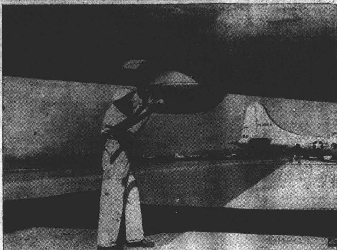
SUPERFORT'S NEW TURRET —New lower rear turret on the Boeing B-29 superfortress, which is remotely controlled and does not house the gunner as in the original fortress.
