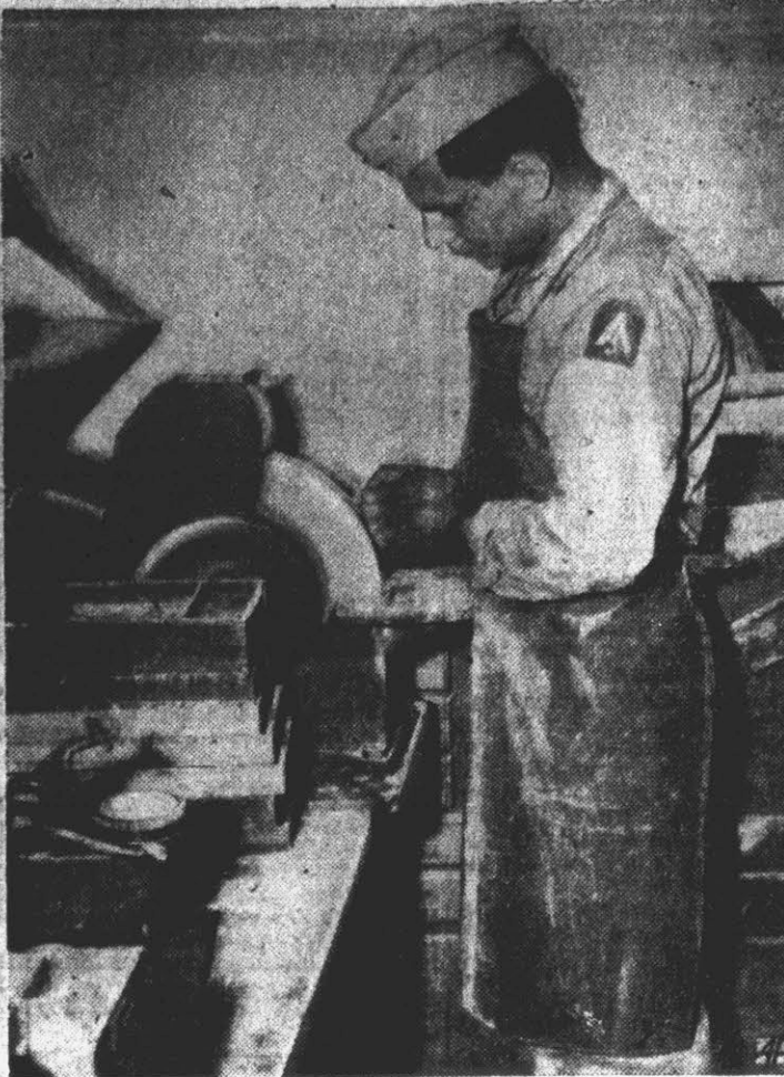
MOBILE CLASSES UNIT—Pfc. Edward Schmaldest of Allentown, Pa., grinds an optical lens to fit a prescription in his workshop with the 12th medical supply mobile optical unit at a Fifth Army base in Italy.
