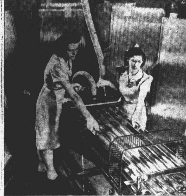
'DRY CLEANING' TUBES—Five-foot-long glass tubes for 100-watt fluorescent lamps for war plants get a "dry cleaning" from this brush and suction cleaner in the Westinghouse lamp division plant at Fairmont, W. Va.
