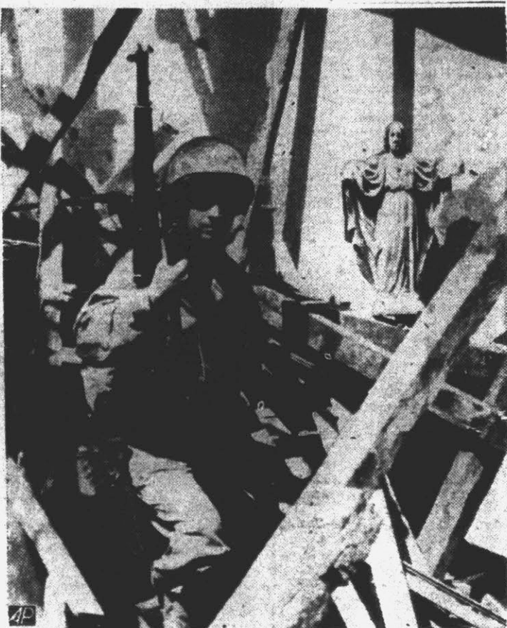
Marine Sgt. Carroll J. Willford of Route 1, Mooreville, N. C., stands amid the debris of a Catholic chapel in the village of Nagas on Asan Beach, Guam. The chapel with walls two feet thick, was wrecked by the pre-invasion bombardment. The statuette of Christ, however, remained upright on the altar, although it was nicked and one hand was knocked off. (AP Photo from marine corps).
