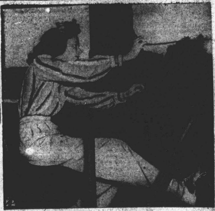
GIRL ENGINEER —Altha Fay Ellis, 29, Corsicana, Texas, operates controls of 20-ton gasoline locomotive at Army Air Forces training command station at Randolph Field, Texas. Locomotive handles oil cars on field.
