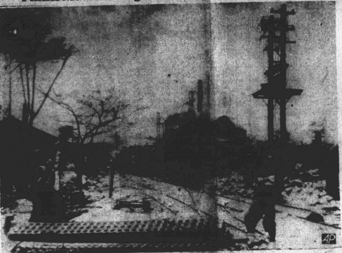
U. S. soldiers probe the ruins of the Japanese sugar refinery on Saipan Island in the Marianas after the successful landing on June 14. Aerial bombing left the refinery shattered and burning. (AP Wirephoto from Signal Corps).
