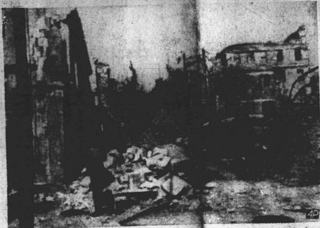
The caption accompanying this picture, transmitted by radio from Moscow, says it shows the damage inflicted on Lenin street, the main thoroughfare in Sevastopol, in the German retreat. (AP Wirephoto via Radio from Moscow).
