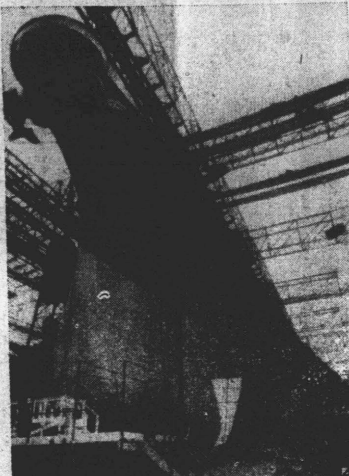
The 45,000-ton battleship U. S. S. Missouri lowers on the Brooklyn Navy Yard ways as she awaits her launching scheduled for Saturday. Under construction since June 6, 1941, the Navy calls her the "World's mightiest battleship." (AP Wirephoto.)
