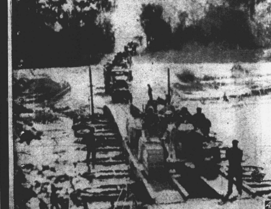
Rumbling across a pontoon bridge built by U. S. army engineers, this line of heavy American artillery, drawn by tractors, moves up to the front as Allied forces expand their territory from the Salerno bridgehead in Italy. This Army Signal Corps picture was radioed from Algiers.
