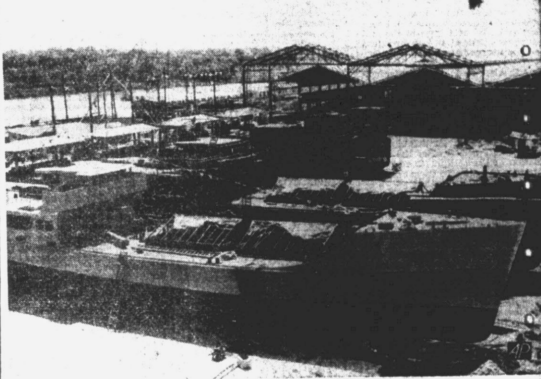
Poised in the foreground just before launching stands the first of 100 "assembly line" cargo ships for the army being built at yards of Higgins Industries, Inc., at New Orleans. Behind are parts of similar ships, which are constructed on movable ways, taking shape as they move toward the water. When one is launched, the next moves into its place. The first was launched 88 days after the contract was awarded. The ships are 170 feet long.
