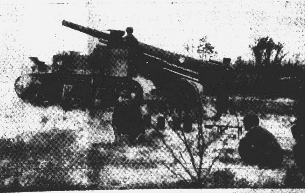
ARMY M-12 IN ACTION—A 155 mm. gun, mounted on the new U. S. Army M-12 gun motor carriage, is fired at Aberdeen, Md. The M-12 does 30 m.p.h. over rough terrain.
