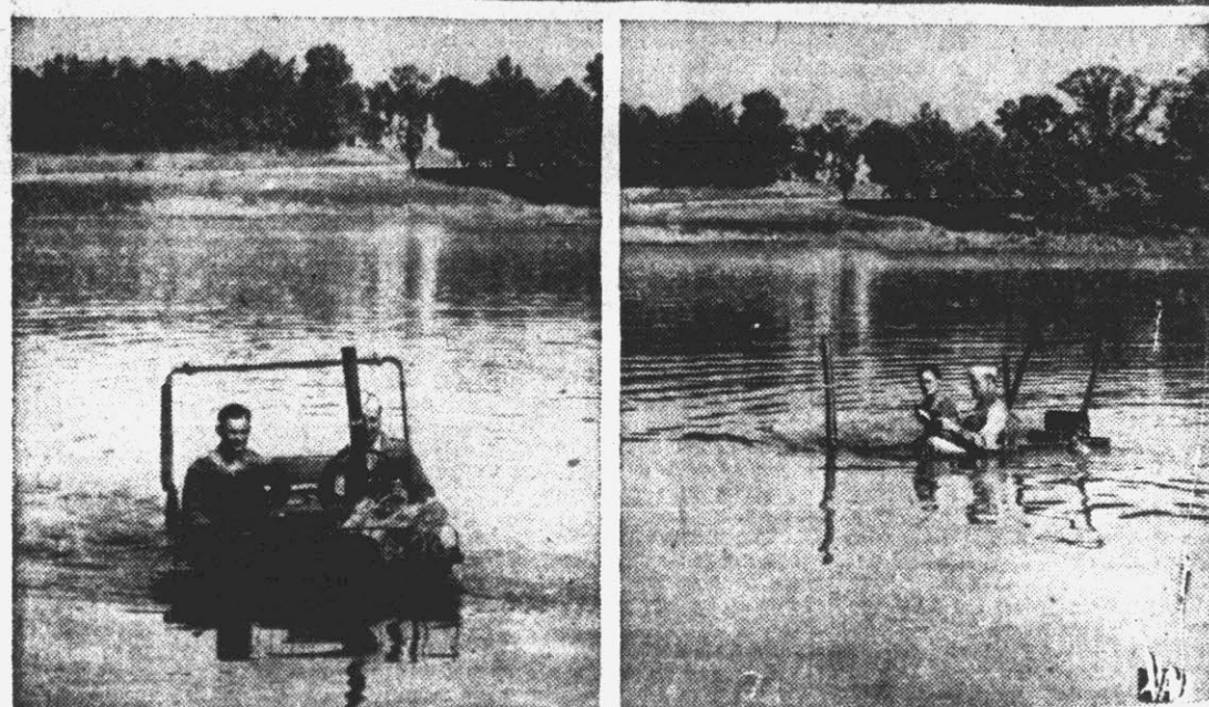
That very versatile vehicle, the Army jeep, with a few construction changes and waterproofing of the motor and vital parts, in a demonstration at Sparanburg, S. C., proves its ability to navigate, almost submerged in shallow water. (At top) Capt. John J. De Rosa of Long Island, N. Y., who directed changes at nearby Camp Croft in the necessary changes and preparations, heads the jeep towards the water. (At bottom) Capt. De Rosa, with Lieut. William F. Williams of Olean, N. Y., as a passenger, "tours" the lake bed and (at left) leads for shore after the demonstration. Note vertical exhaust pipe. (Signal Corps Photo.)
