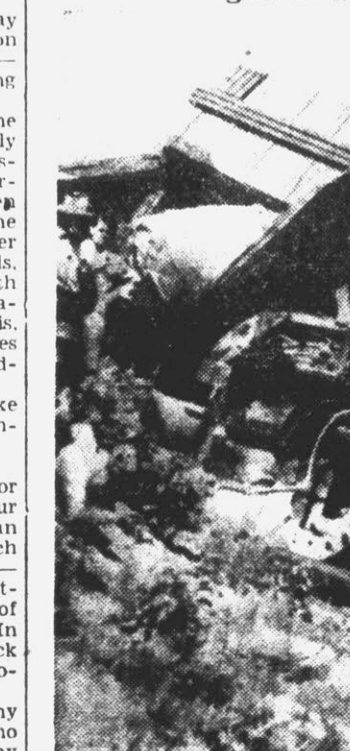
Three trainmen were killed and three were injured in this pile of wreckage resulting from the head-on collision of two Seaboard railroad freight trains at Garlington, a flag stop near Clinton, S. C. The wreck occurred June 1.
