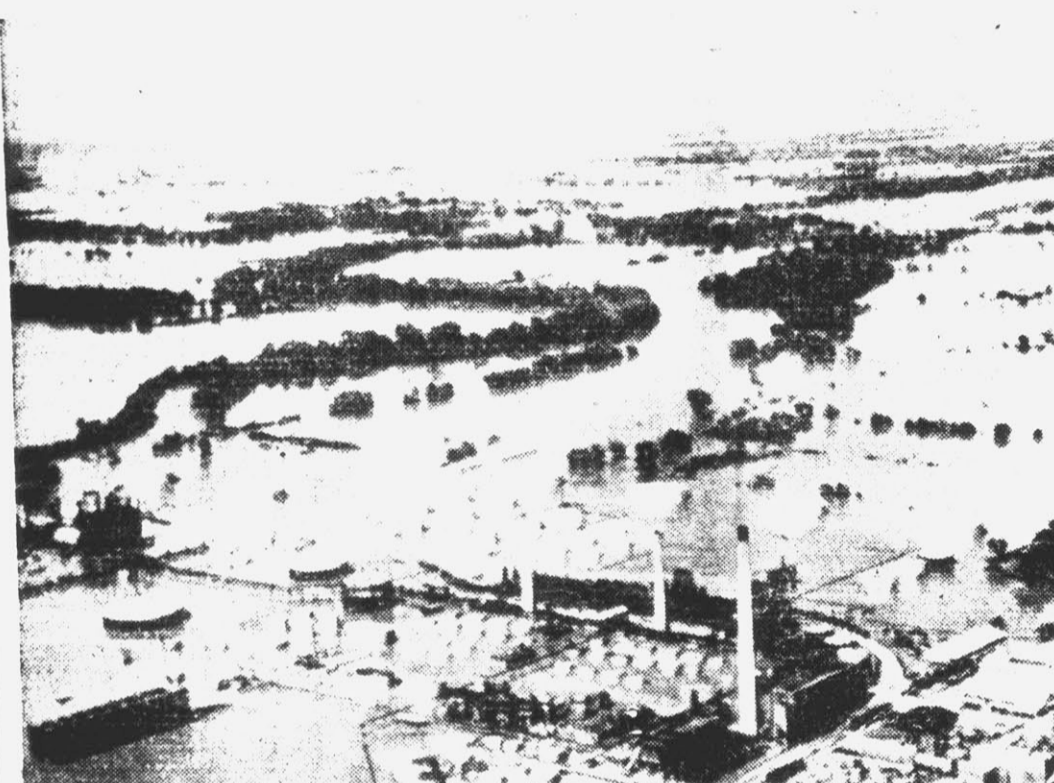
The National Refinery Co., northeast of Coffeville, Kans., was flooded by high water from the Verdigris river in the flood area of Kansas. (Associated Press photo from U. S. Army Air Force.)
