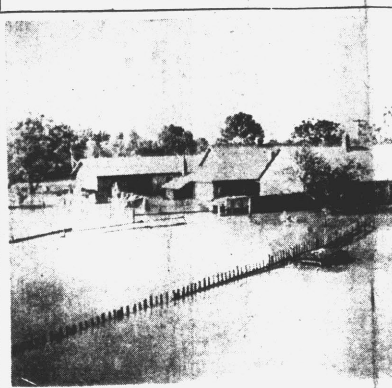
These homes at Pine Bluff, Ark., stand close to the Arkansas River levee (right)—but not close enough. So they were flooded by backwater from the swollen stream. A family automobile was left behind when higher ground, and only the top of the car remains above water. (Associated Press photo from U. S. Army Engineers.)
