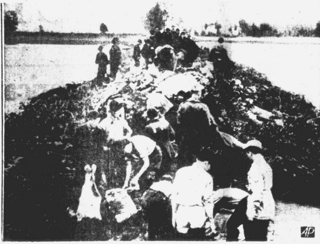
Identified by the large letters "FW" on their blue fatigue clothing, these Axis prisoners of war of undisclosed nationality here work under supervision of U. S. Army Engineers at filling a break in the Mississippi river levee near Ste. Genevieve, Mo. The faces of the men were painted out in the picture at the request of the Army engineers. They were put to work fighting flood waters by emergency authority.
