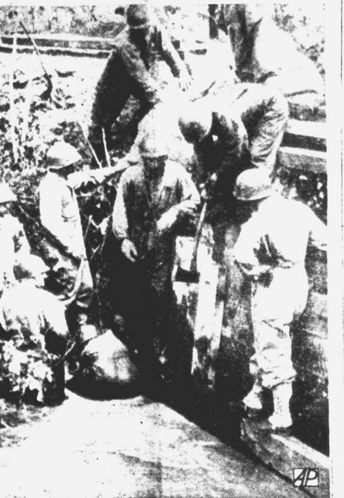
Soldiers from Camp Chaffee's Fourteenth Armored Division were in the thick of the fight against a record-breaking Arkansas river flood at Fort Smith, Ark. This official U. S. Army Signal Corps photo shows a unit "locking up" a sluiceway to prevent backwaters from washing out of U. S. Highway 71, a mile from the Van Buren-Fort Smith bridge.
