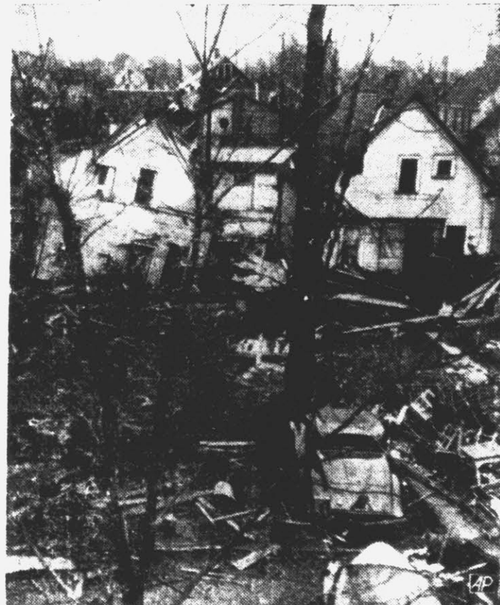
This was a typical scene of damage in scattered sections of Cleveland, Ohio, after a tornado swept the east and west sides of the city. Some homes were twisted from foundations, other were unroofed, and scores of garages were splintered. The twister struck in several sections of northeastern Ohio. Two children were killed near Medina, about 150 were injured in other places and nearly 2,000 homes and several war plants were damaged.
