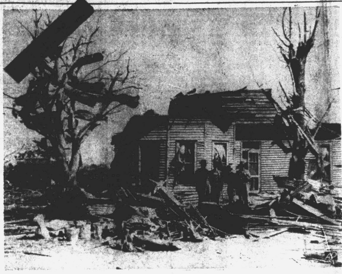
Here are the remains of one of the numerous buildings wrecked by a tornado that struck Hackleburg, Ala. At least four persons were killed and 50 injured, Mayor C. E. Fell estimated the damage at $500,000.
