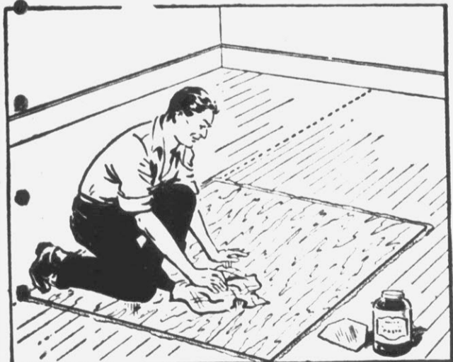
FIRST THE DESIGN IS LAID OUT AND SQUARES ARE PASTED DIRECT TO FLOOR.
