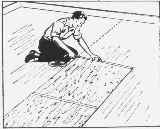
FEATURE STRIPS ARE FITTED ALONG EDGES OF SQUARES AND PASTED DIRECT TO FLOOR.
