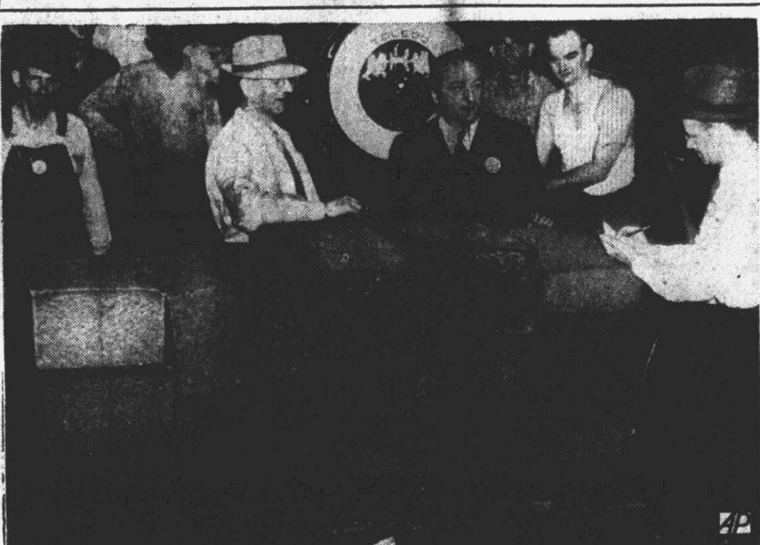
The first bales of synthetic rubber produced at a U. S. government-owned plant at Baton Rouge, La., are here being weighed—less than five months from the time ground was broken for construction of the plant. Participating in the ceremony are W. A. S. Harmon (with arm on bales), project engineer for the Firestone Tire and Rubber Co.; Guy E. Panero (in dark coat), project engineer for H. K. Ferguson Co.; and A. M. Ives (right, checking weights), superintendent for Blaw-Knox Co.
