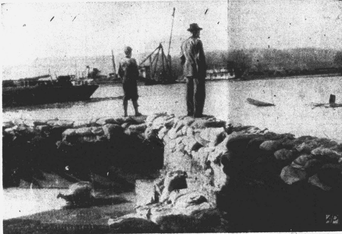
Topped by sand bags, the great five-mile wall of concrete has saved the industrial city of Portsmouth, Ohio, from a disastrous flood once more. A man and a boy stand atop the sand bags and watch the surging water. The flood water on the Ohio river rose to 66.9 feet, just 1.1 feet under the top of the 62-foot dike. The same wall saved the city in the great flood of 1936.
